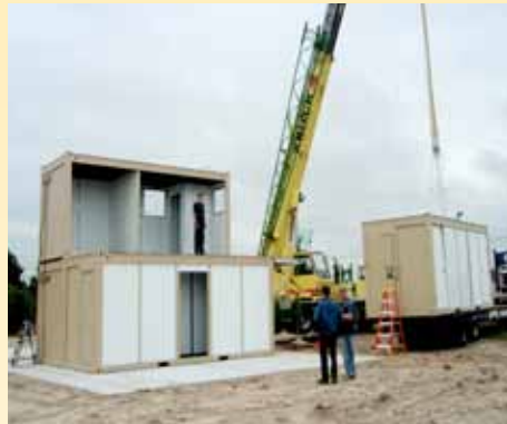
Cubic is partnering with UXB International, Inc. on a modular training facility called RATPAC™ that can be reconfigured. Cubic is providing the technology, such as special effects and videotaping for after-action reviews.
